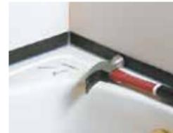
Factory installed nailing flange
